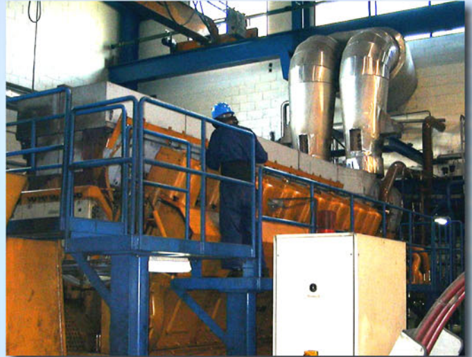
Maintenance on a Caterpillar® 16CM32 engine
