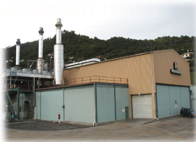
Grenlec-Quenn's power plant in St. George, Granada generating 18.4 MW.
